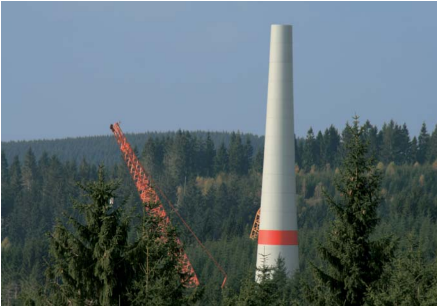
Hilchenbach: Tower construction with a 600 ton crawler crane.
