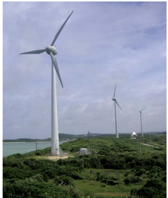
Karimata, Miyako Island: three out of four E-44 turbines.
