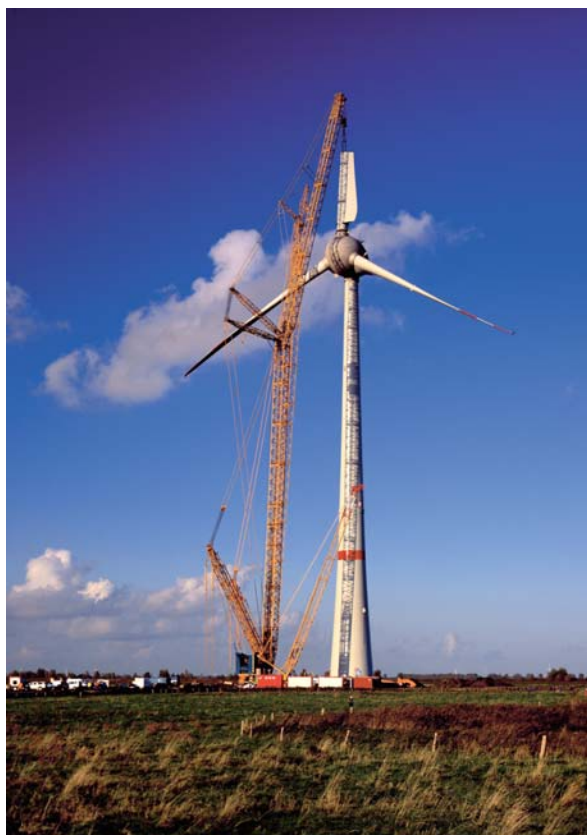
Mounting steel segment of third rotor blade.
