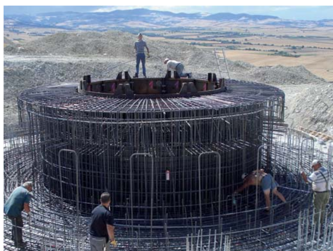
Foundation work for one of 13 E-82/2 MW turbines.
