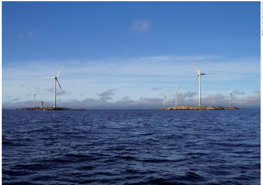
With an average wind speed of 9.4 m/s (at 65 m hub height), Båtskär is an ideal site for wind energy use.
