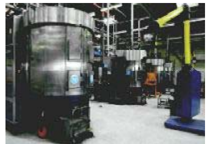
Recycling of wire saws and the sludge they produce can help to minimize the waste from silicon PV plants PHOTOWATT INTERNATIONAL;
